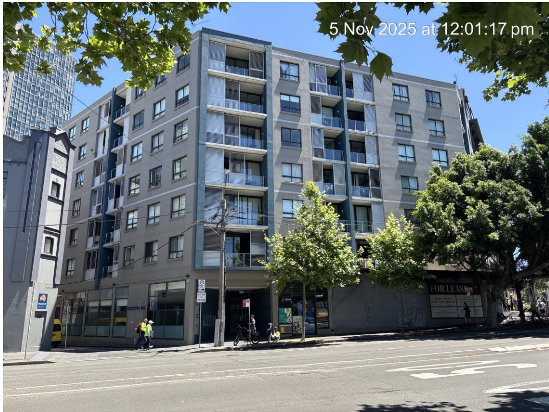
Figure 1: 49-53 Regent Street, Chippendale, viewed from the south-east
